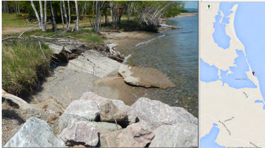
Figure 20 Heavy erosion just north of revetment – Melikewe’j.
